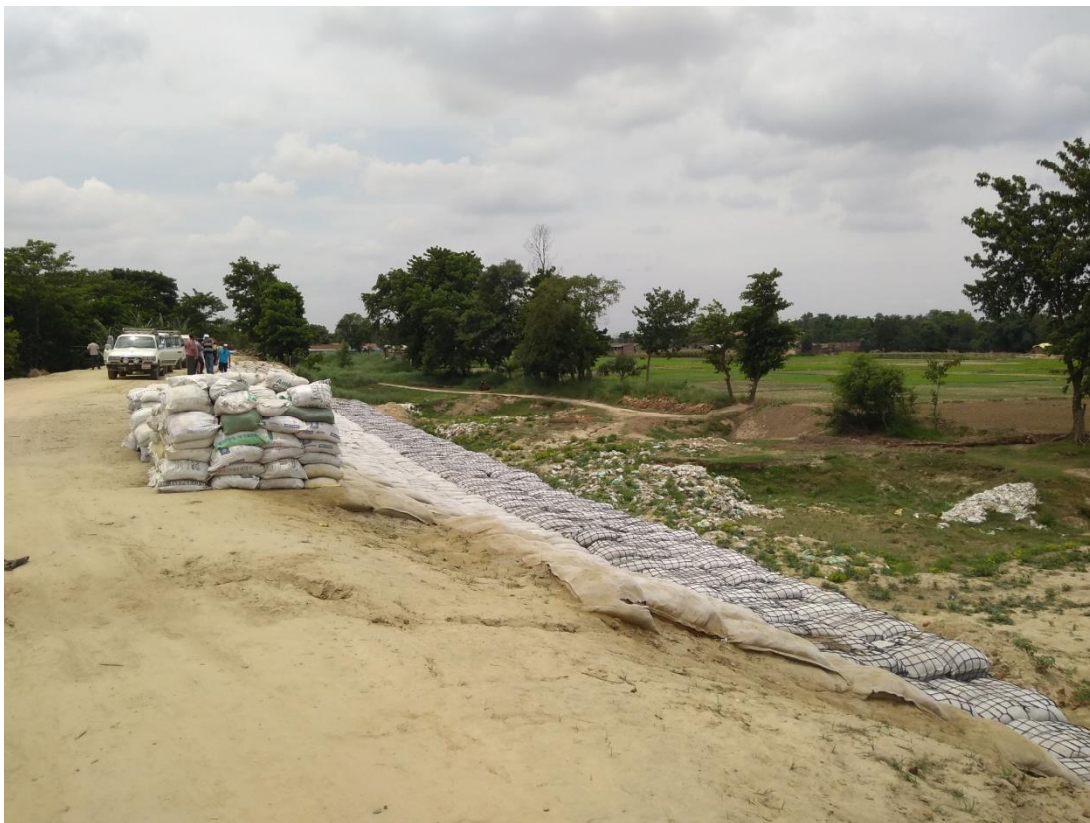
Fig.-6.4: Embankment protection work near Banjaraha village Nepal
