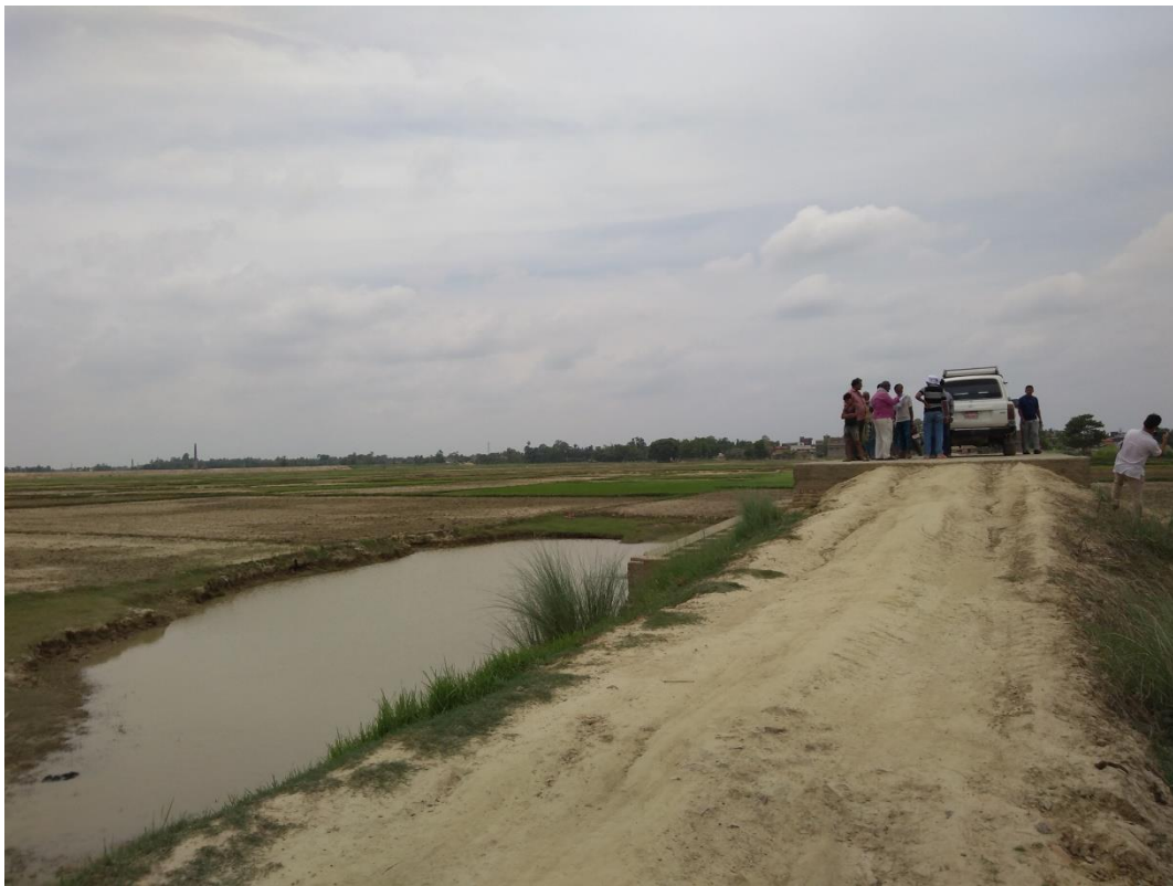
Fig.-6.2: Existing Culvert on Guhabari-Bhawanipur road in India
