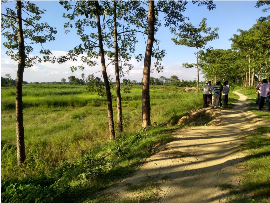
Fig.-5.1: Jamindari Embankment in India near Bara-Udhoran village, Nepal
