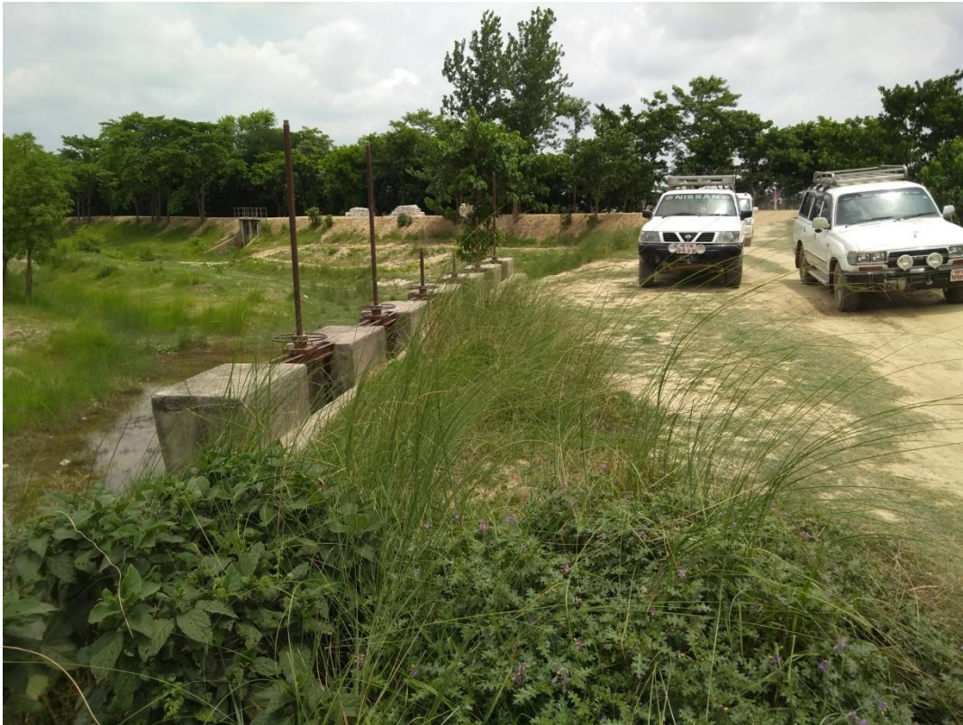
Fig.-6.1: Gated AFS on Lalbakeya Right Embankment near border
