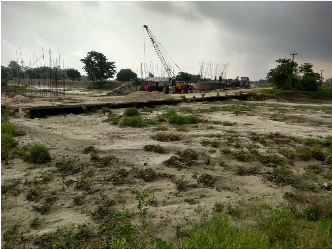
Fig.-1.5: Construction of Road bridge on Khando river in Nepal
