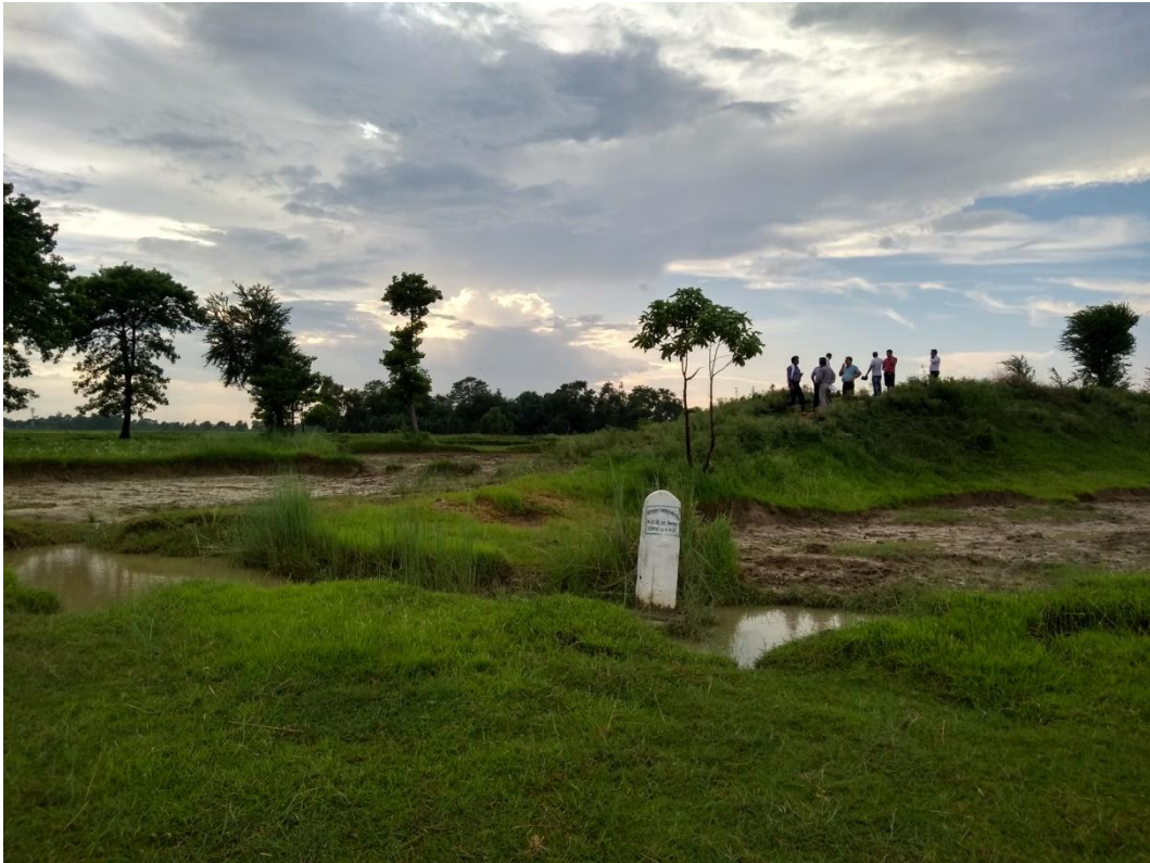
Fig.-2.1: Gap after Zero RD of Kamla Left Embankment near No-man's land
