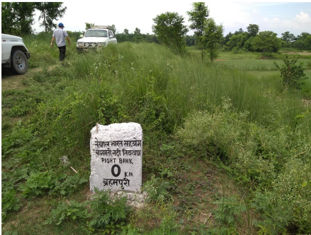
Fig.-7.1: Zero RD of Bagmati Left Embankment in Nepal portion
