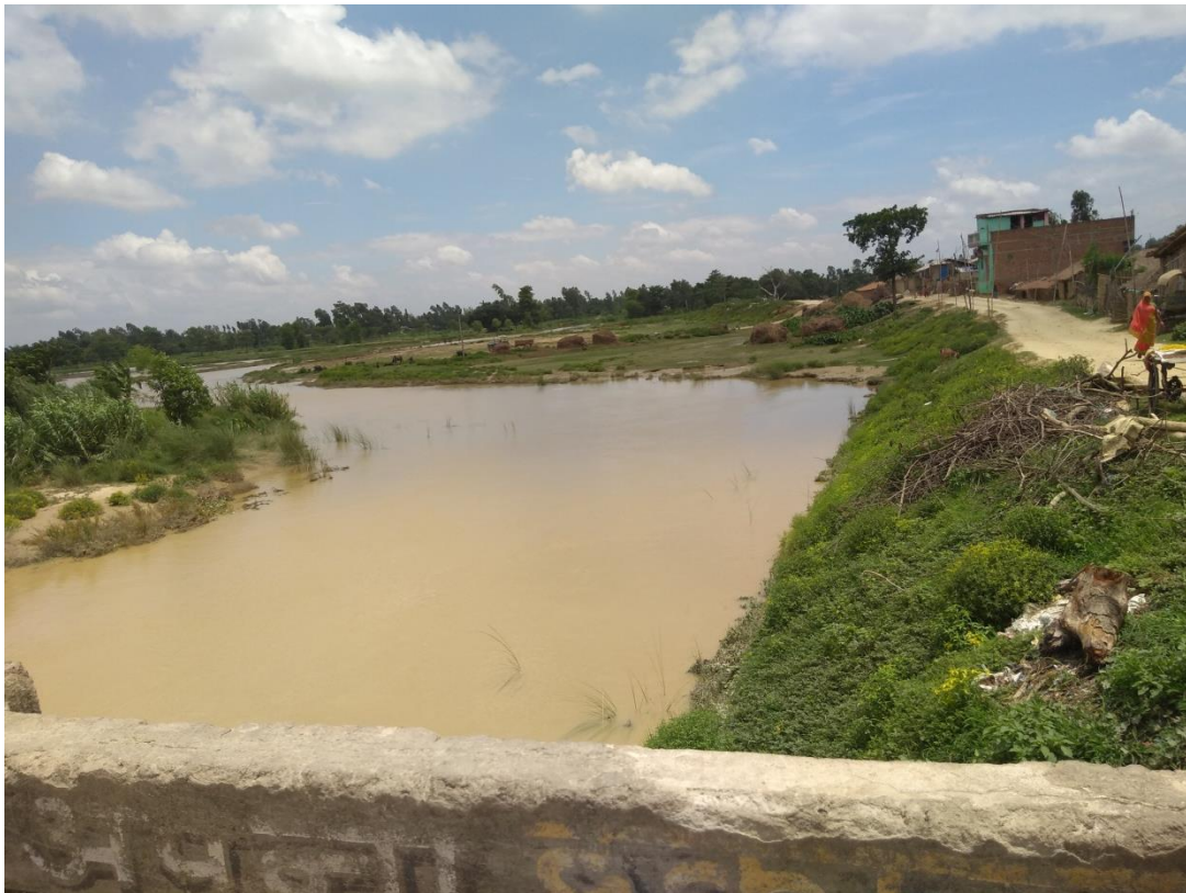
Fig.-4.1: Rato Left Embankment near Bhattamore-Sitamarhi road
